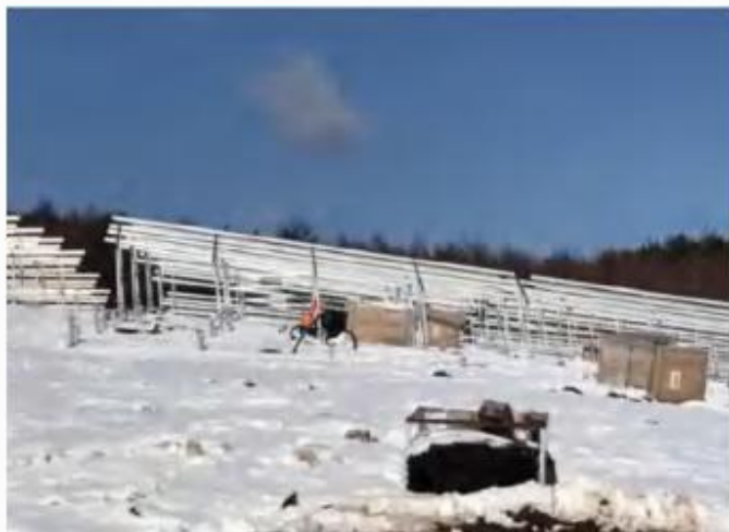
2 Mwp in Japan
